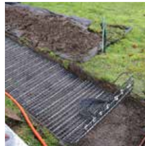
3. Laying the cut to size
